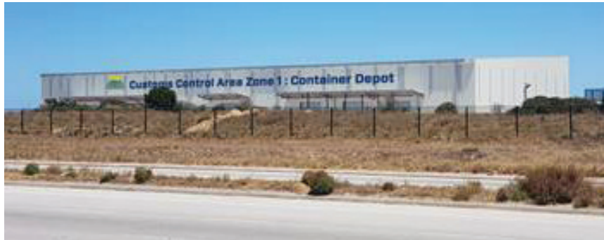
THE Coega Customs Control Area 3,600m 2 warehouse.
