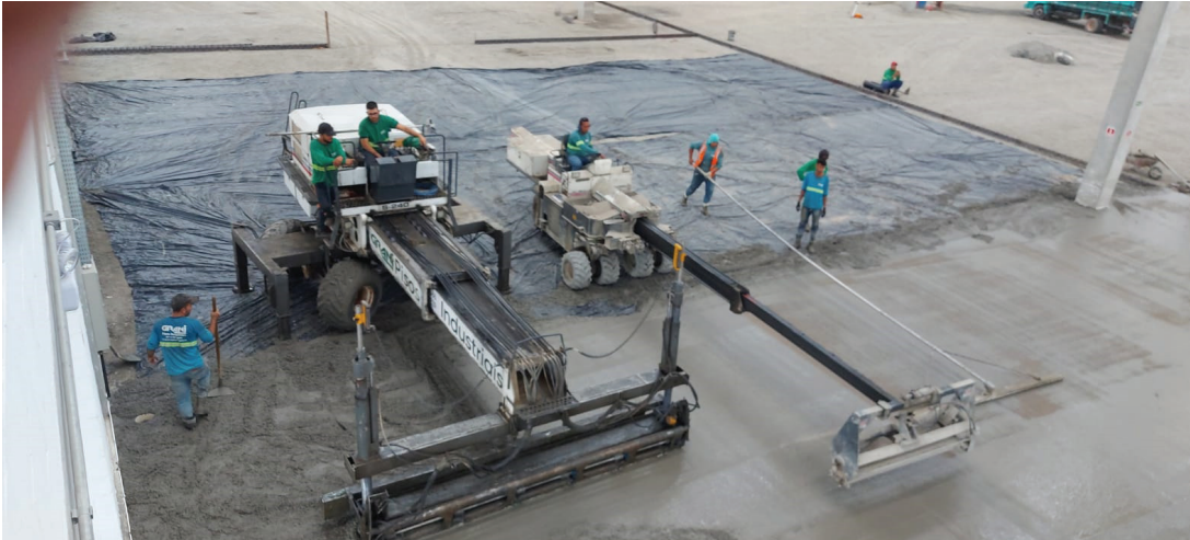
Laser screeding and shake-on happening together.
