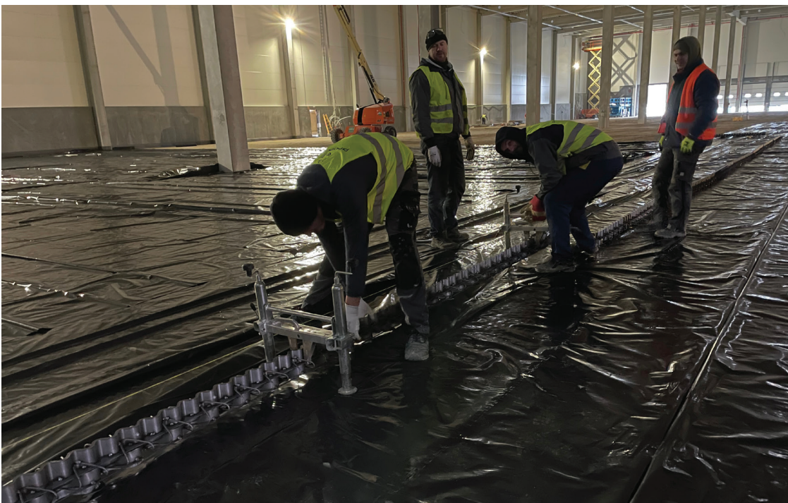
An example of joint preparation with plastic sheeting, ready for pouring.
